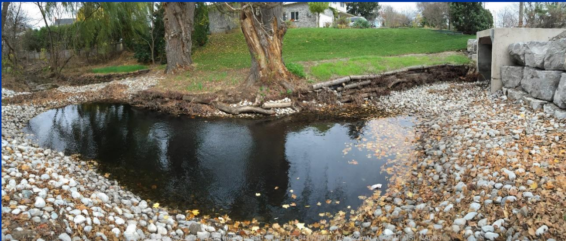
Plunge pool and vegetated crib wall at embedded culvert outlet.
