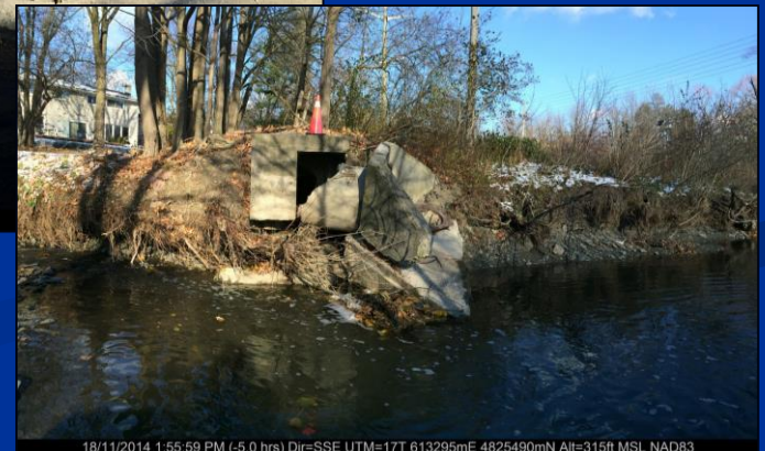
Cooksville Creek, reach downstream of concrete lined channel.
