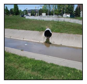
Storm water outflow taken offline with settling pool and vegetative buffer attenuating flows into re-naturalized channel.
